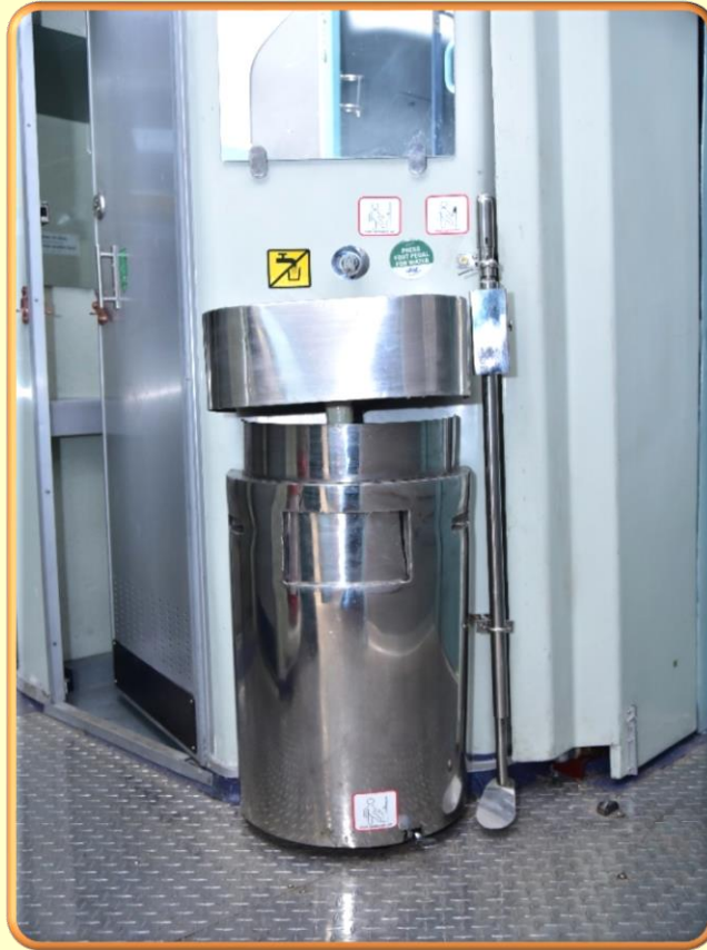
Outside washbasin with foot operated Water tap & Soap dispenser
